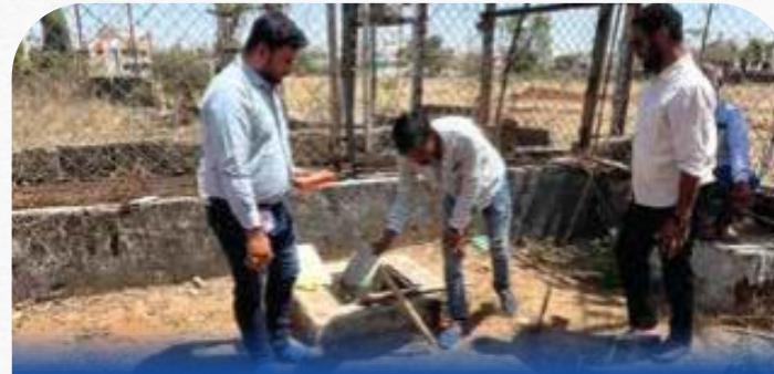
Underground Cable Network Project – Himmatnagar & Idar, Gujarat
