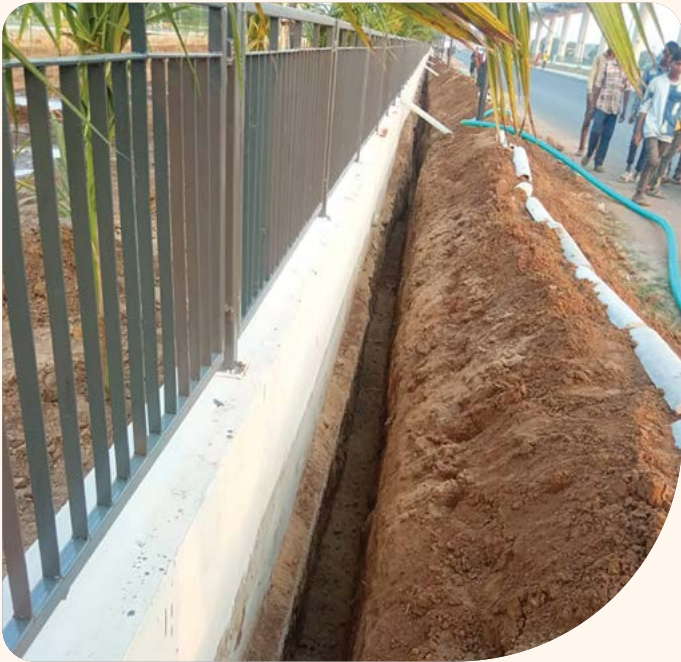
11 kV Underground RDSS Project, Gandhinagar (Government)
