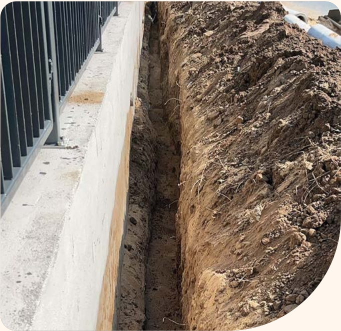
11 kV Underground RDSS Project, Ahmedabad (Government)
